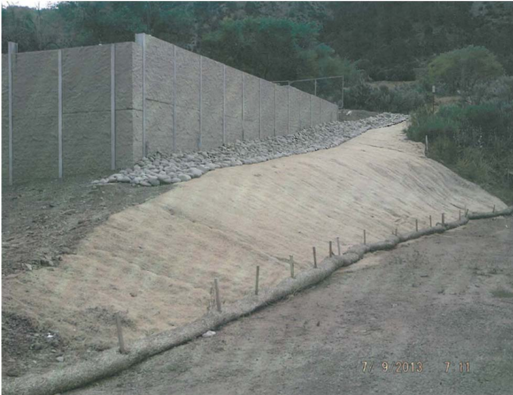
Sos' embankment after RFTA's construction
